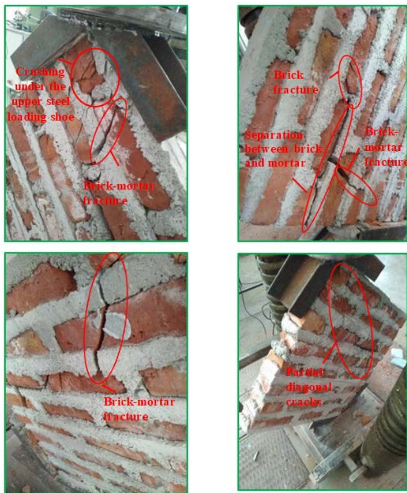
Figure 8. Cracks and failure modes in the MWFM1 samples
