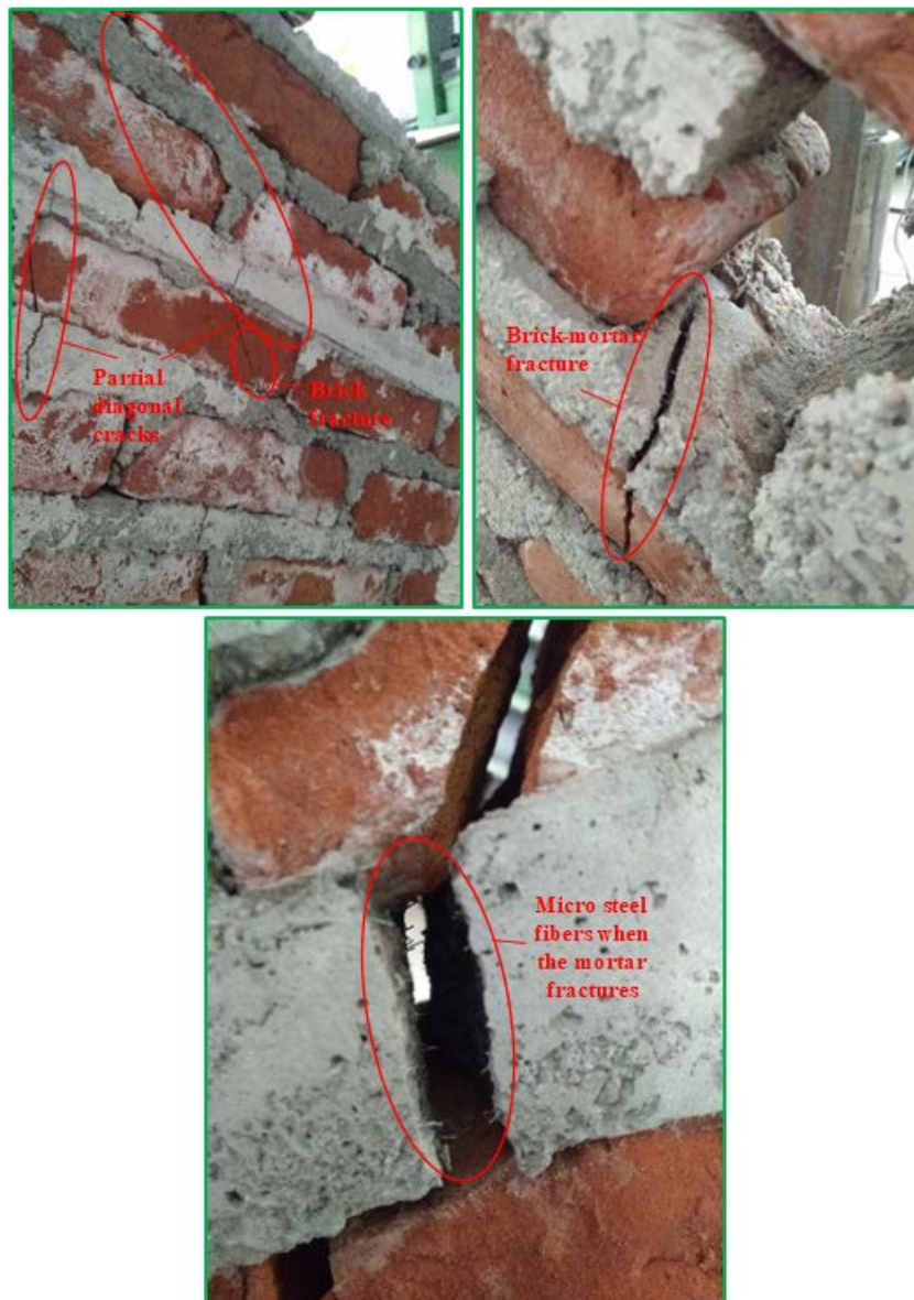
Figure 10. Cracks and failure modes in the MWFM3 samples
